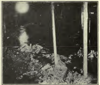
A "damp" cellar
